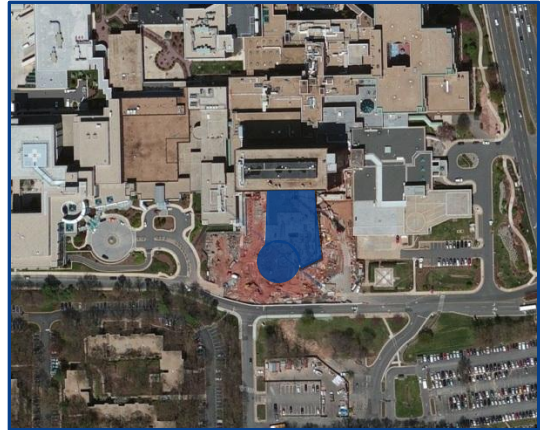
Figure 1: Aerial map from Bing.com showing the location of the building site
