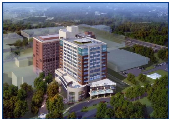
Figure 2: Exterior rendering showing the circular entrance and precast concrete façade (Provided by Turner Construction)
